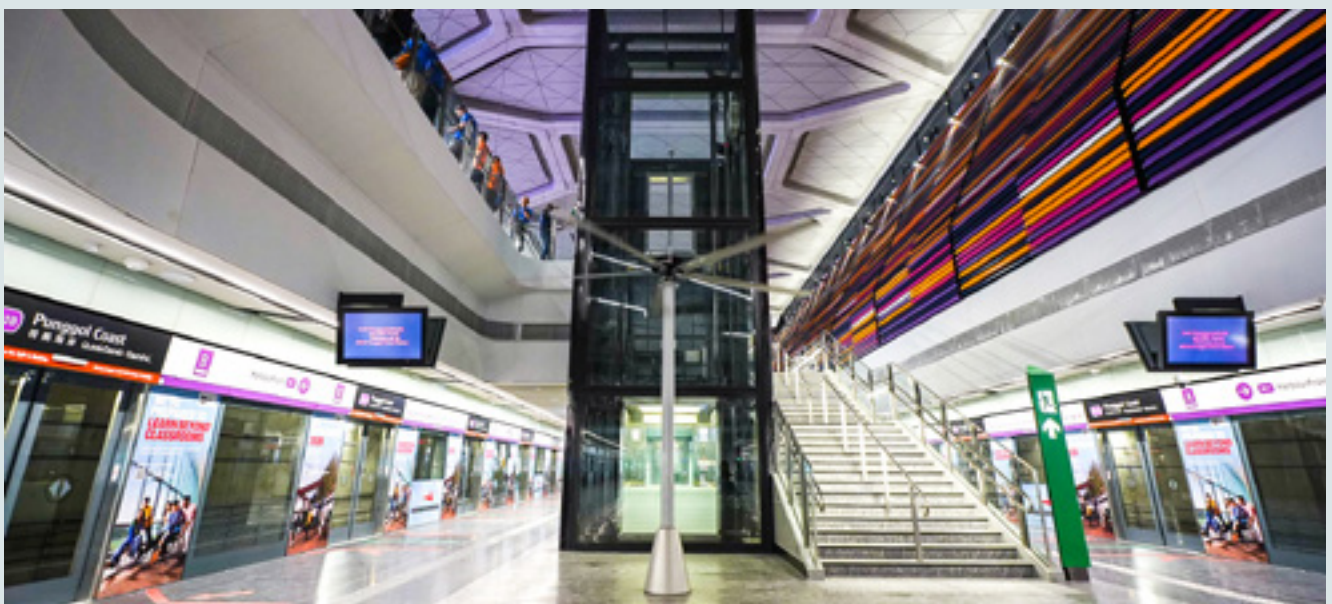
Hybrid fans at the platform are used in conjunction with the Punggol Digital District's District Cooling System to keep the station feeling cool while utilising energy efficiently.
